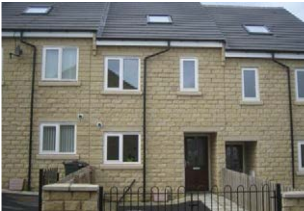
Stamford Brook masonry houses used in field trial
